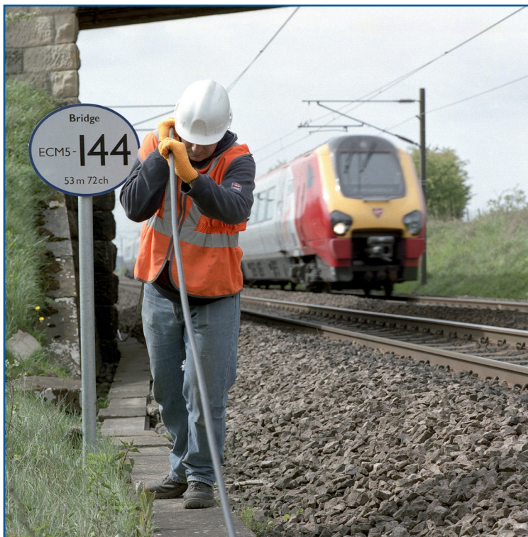
Telecommunications installation by Skanska for Network Rail
