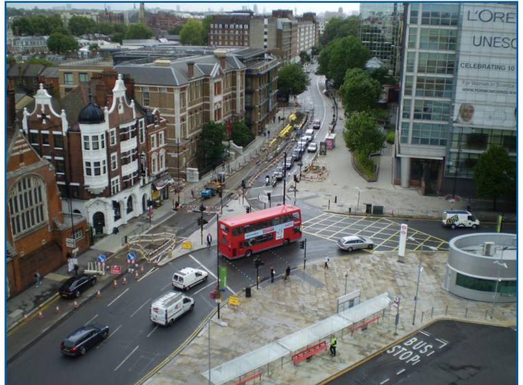
North London Gas Alliance Contract (Skanska)
